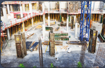
Shuttering Works
